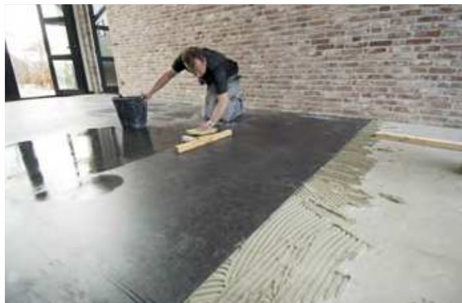
12 Grouting and cleaning 12 Rejuntado y limpieza
