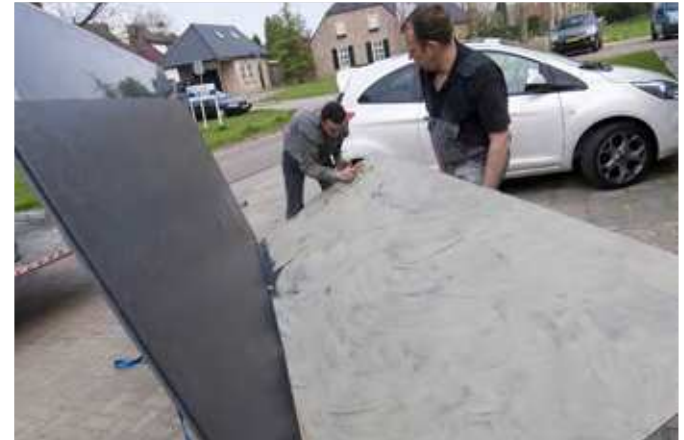
05 Fully gluing of the slab 05 Encolado completo de la tabla
